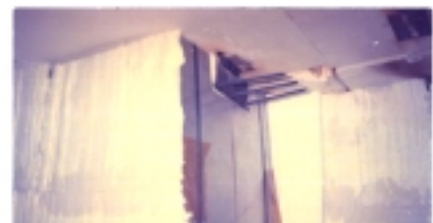
ALTRA ® Modules Installation SKA50 anchors and steel compression plates
